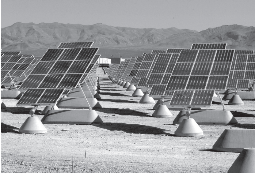
Figure 12.1. Solar photovoltaic array at Nellis Air Force Base, in Nevada, USA. Since all the panels have a similar orientation, the reflection will be concentrated in one particular direction. This particular array uses single axis trackers turning about a roughly polar axis. Credit: U.S. Air Force photo by Senior Airman Larry E. Reid Jr.
