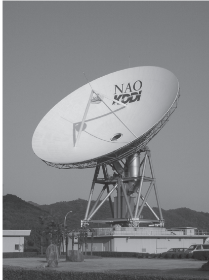
Figure 8.4. The 32 m single dish of Yamaguchi University.
