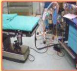
Figure 9.7. Loose cords and cables stretched across pathways in an operating room
