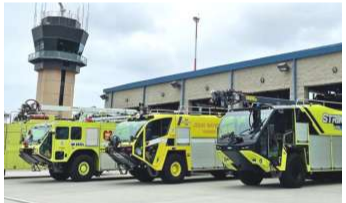
Airport Rescue Fire Fighting Station
