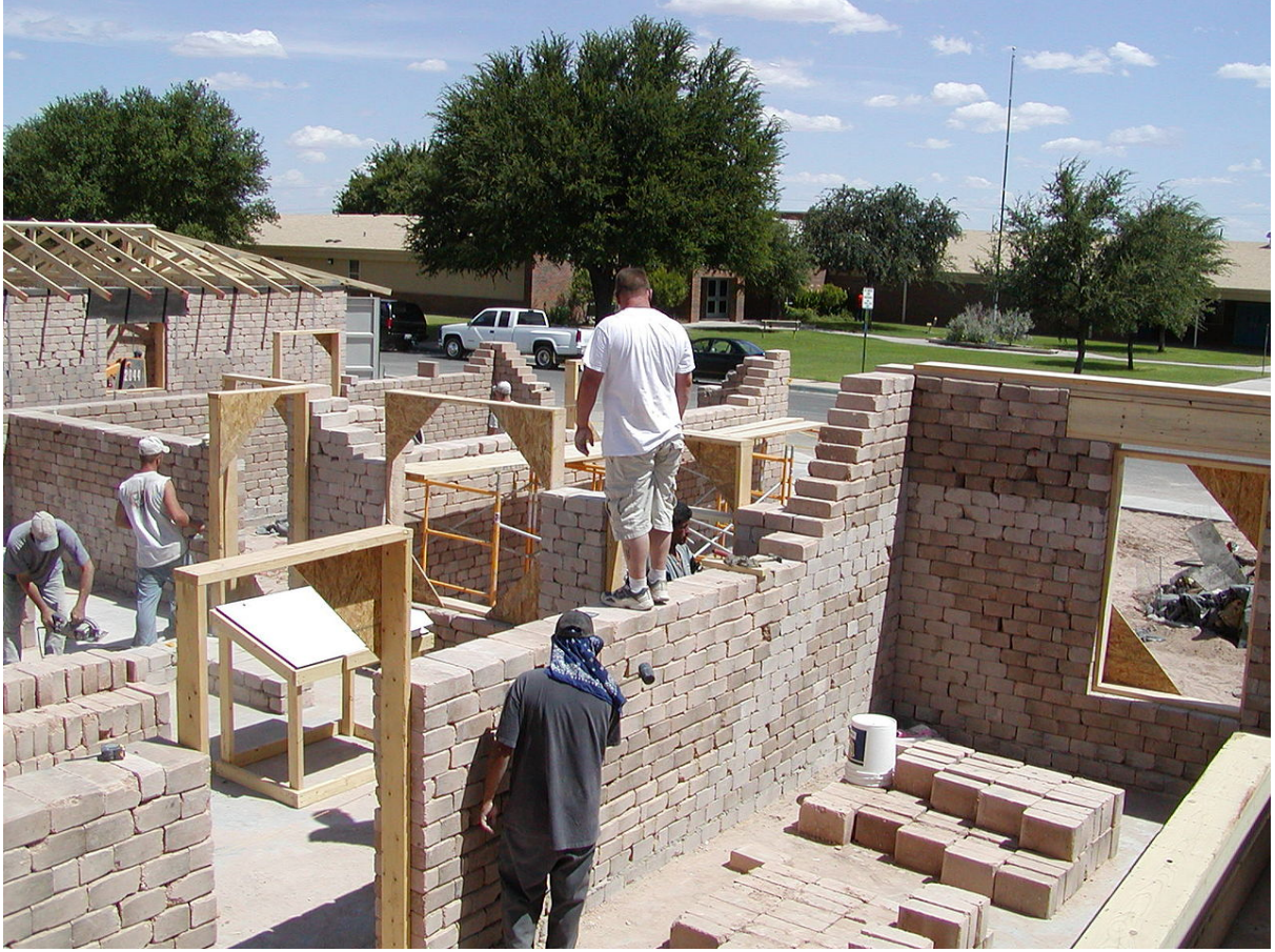
Building a CEB project in Midland, Texas in August 2006
