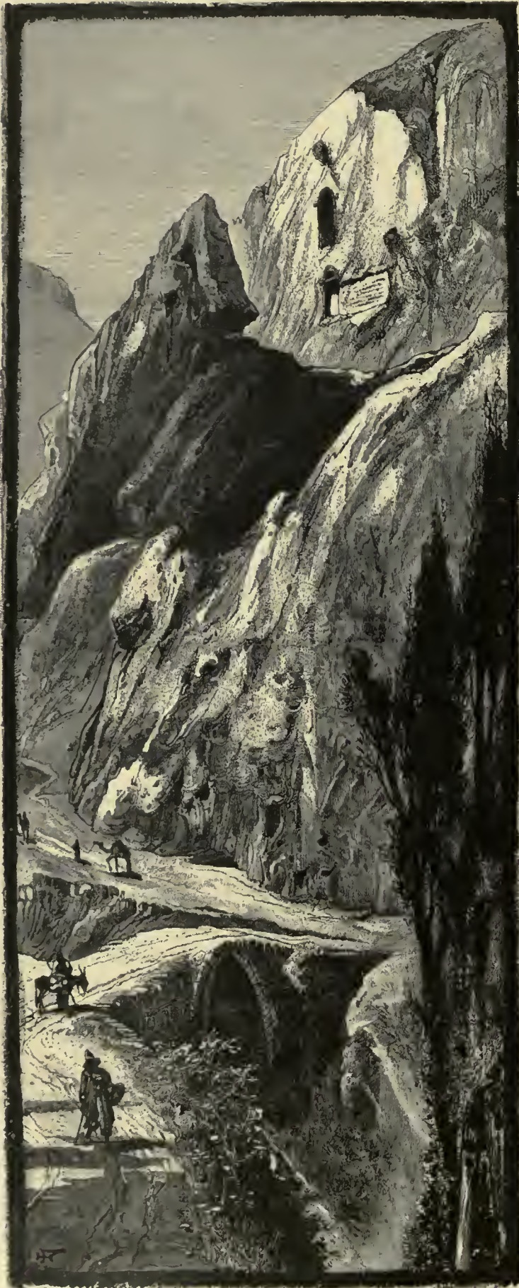
ROAD AND TABLETS CUT IN THE CLIFFS OF WĀDY BARADA. On the north or left bank of the river.
