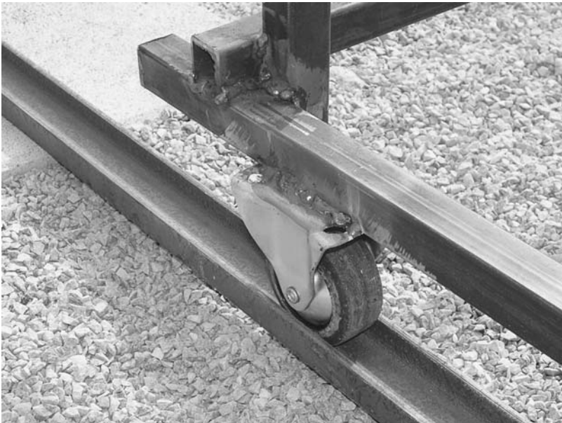
Figure 5.4. Jointing in a welded-steel run-off shed framework.
