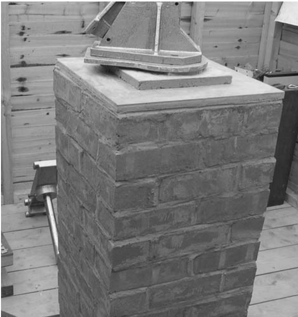
Figure 5.2. Earlier brick pier in my observatory.
