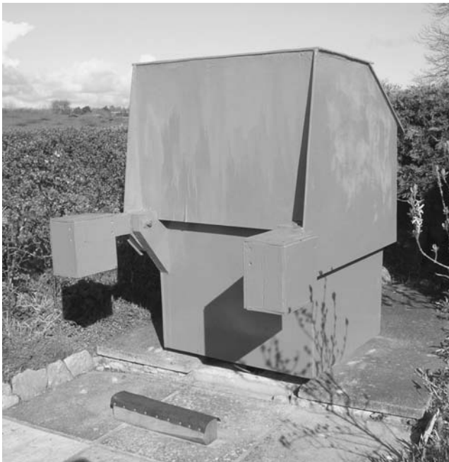
Figure 9.59. View of the counterweight side of the enclosure, the base and the rubber mat on which the upper section rests when the observatory is in use.
