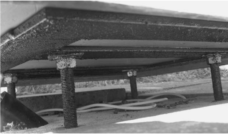
Figure 9.58. Steel baseplate supported on bolts.
