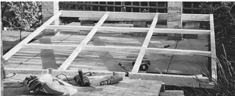
Figure 9.23. Constructing the roof framework.
