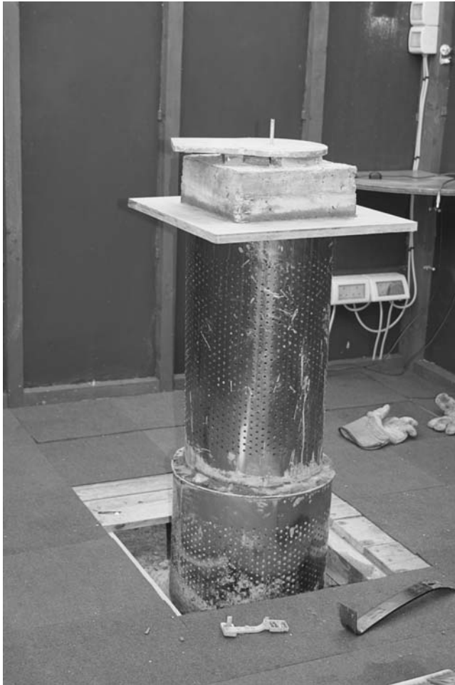
Figure 5.1. Telescope pier in my observatory, cast in concrete in two stainless steel cylinders (bins), with plywood shelf, and aluminium platform set in the top.
