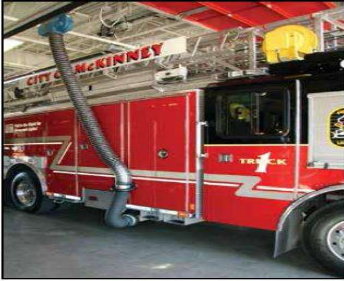
Apparatus exhaust capture systems reduce air pollution in apparatus bays.
