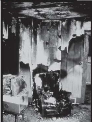
A Typical Conical Fire Pattern
