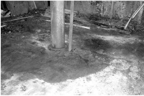
Spalling on the floor
