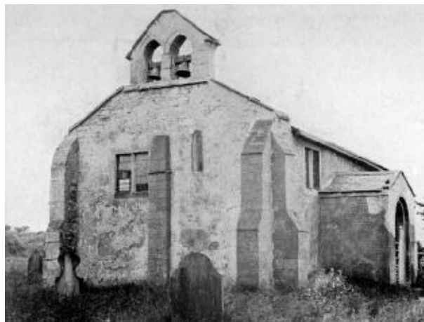
St. Helena's Church in Austerfield, Yorkshire
