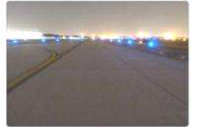
Blue taxiway edge lights
