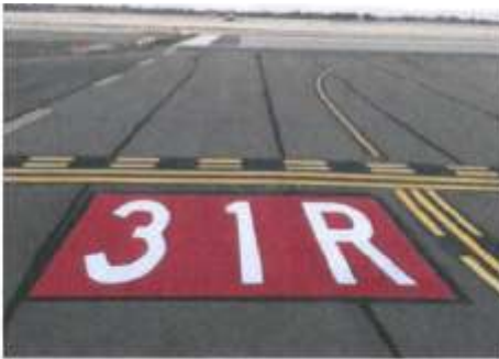
Surface Painted Holding Position Marking
